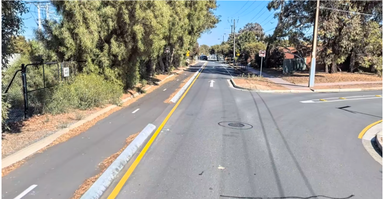
Figure 2: An example of unobtrusive physical separation along the Marino Rocks Greenway.
