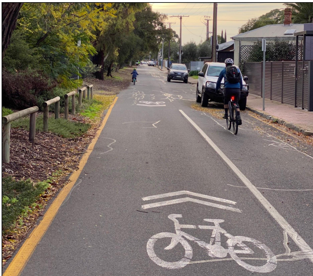
Figure 2: View east along Railway Tce Sth from near the tram underpass.
